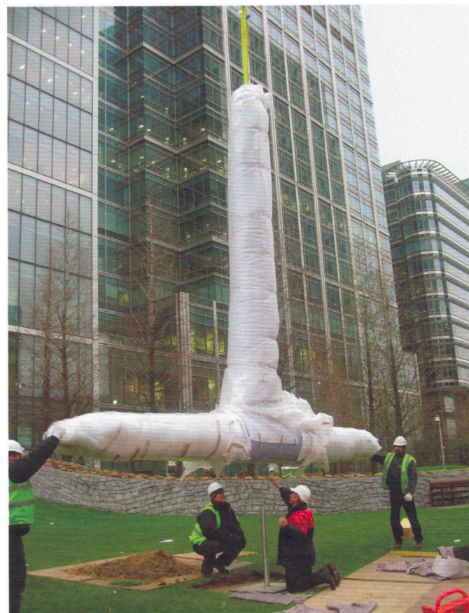
Installing Franz West Verkehrtes T 2006 Over Under : Andrew Sabin, Franz West, Keith Wilson 2007
